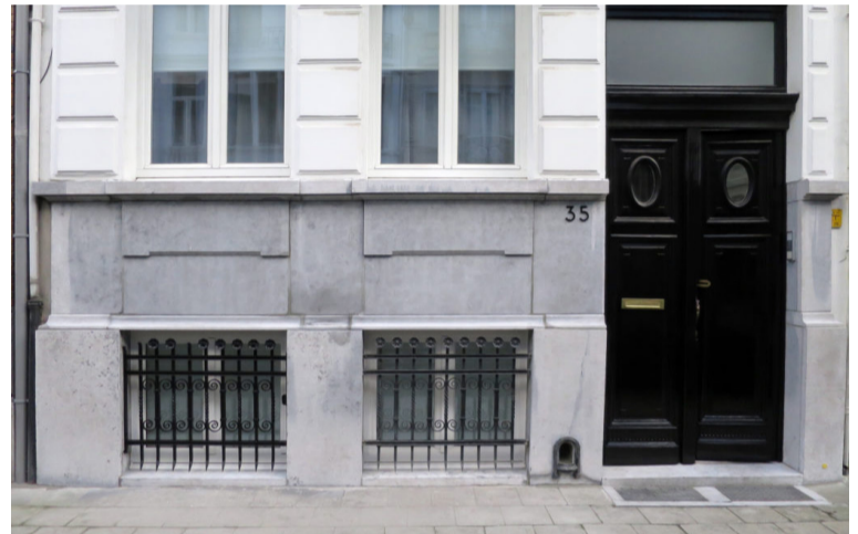
Figure 31: Blue stone (petit granit) used in a façade in Antwerp (Fernandez, 2017).
